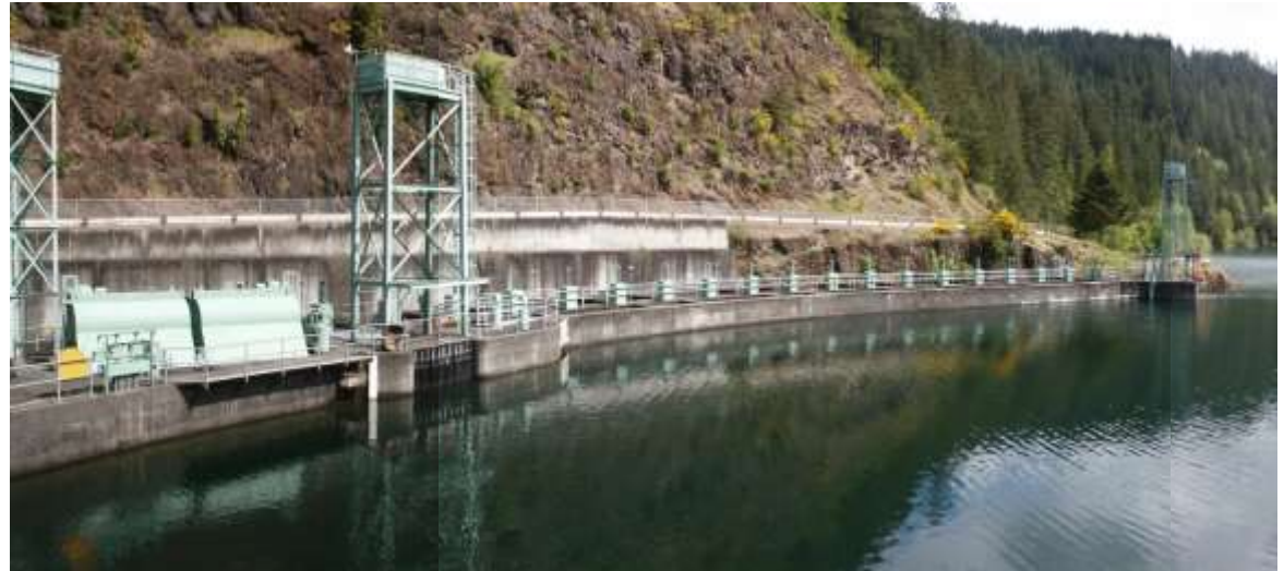
Ladder Exit in North Fork Reservoir Originally Designed for Reservoir Surface Fluctuations up to 6 Meters Current Licensed Operations Limited to 1.5 Meters, and Typically Operated within 1 Meter
