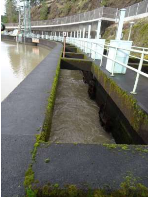
Ladder Exit is Combined with a Downstream Migrant Collector & Bypass System
