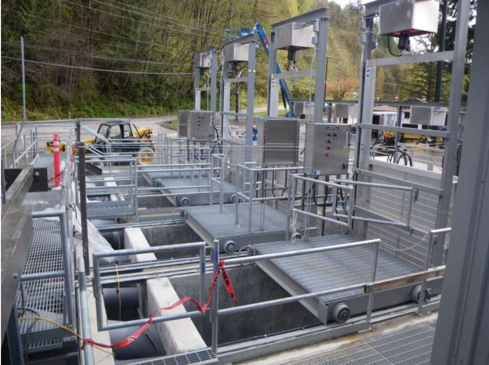
Separate Holding Tanks based on Species and Release Destinations
