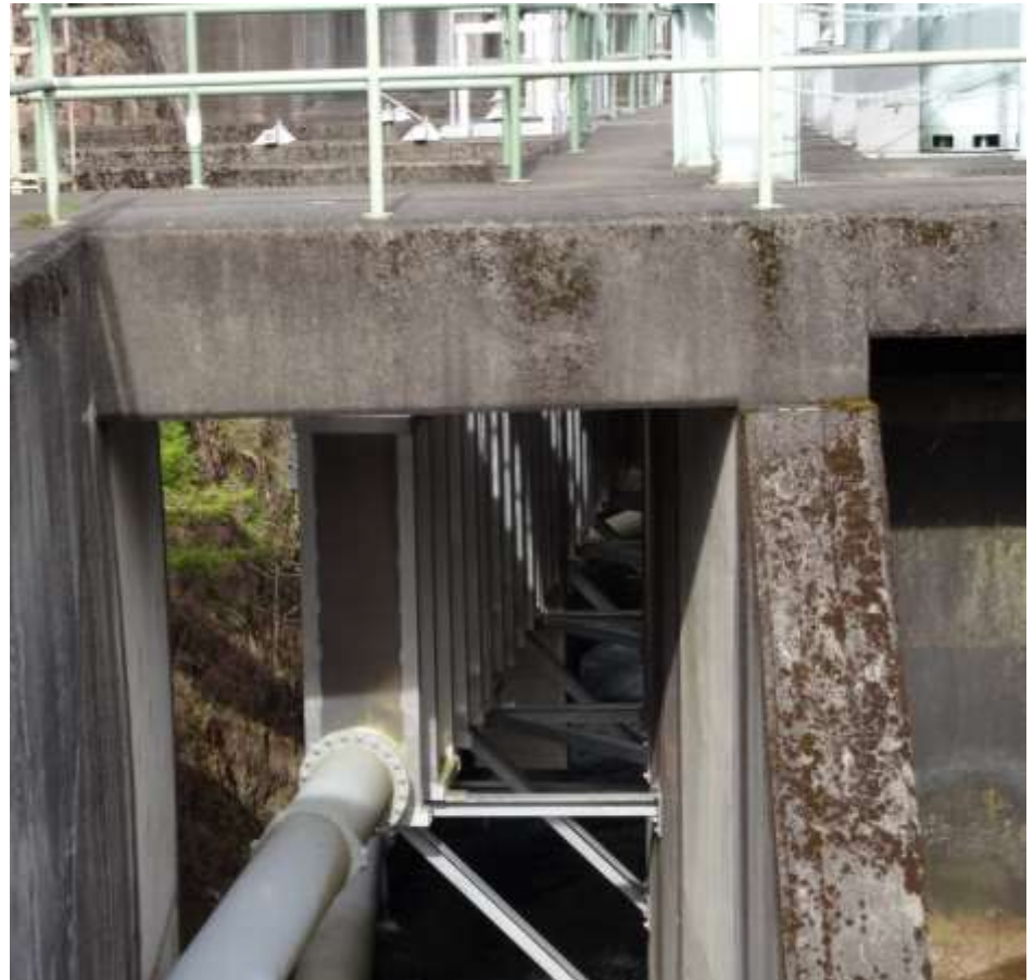
Diversion Box and Pipeline Mounted above Fish Ladder (2011)
