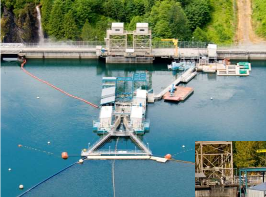
FSC in Ballasted Operating Position
