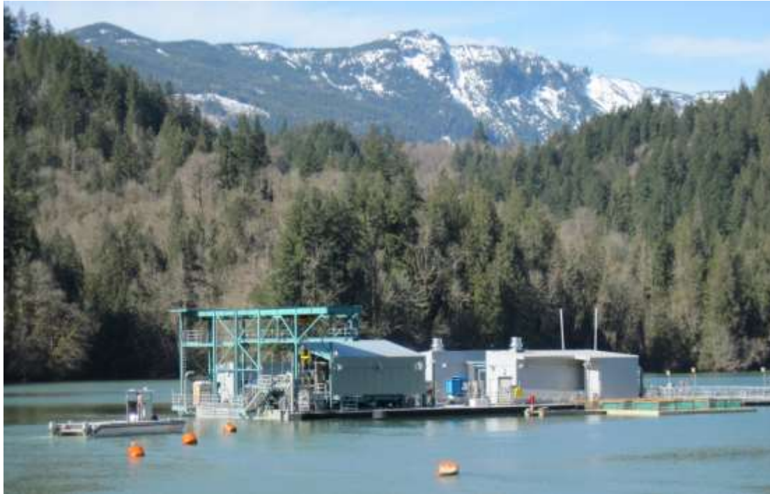
FSC in Ballasted Operating Position
