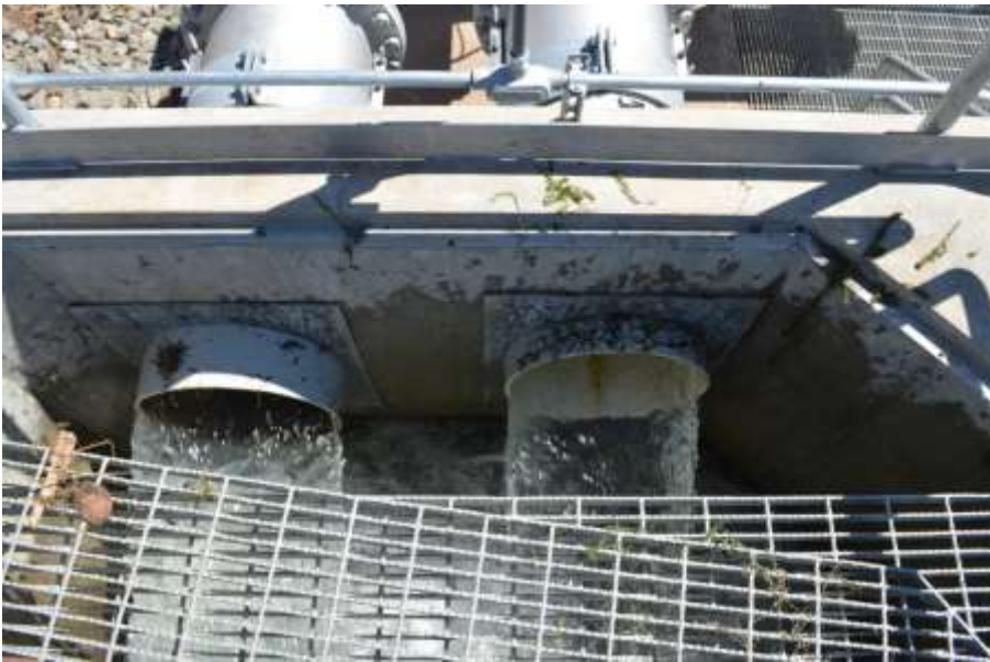
Fish Discharge from Transport Pipes
