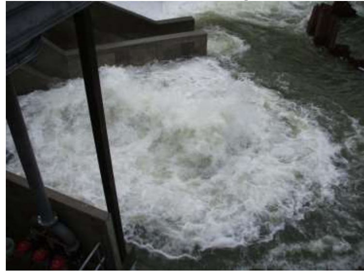
Air-Burst Cleaning Cycle
