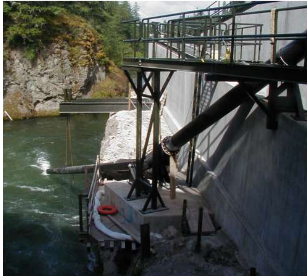
New Hinged Adjustable Discharge (2005)
