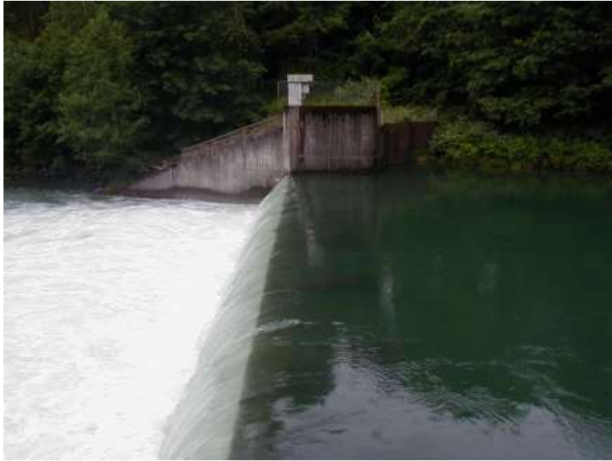
Flow Nappe over Barrier Dam
