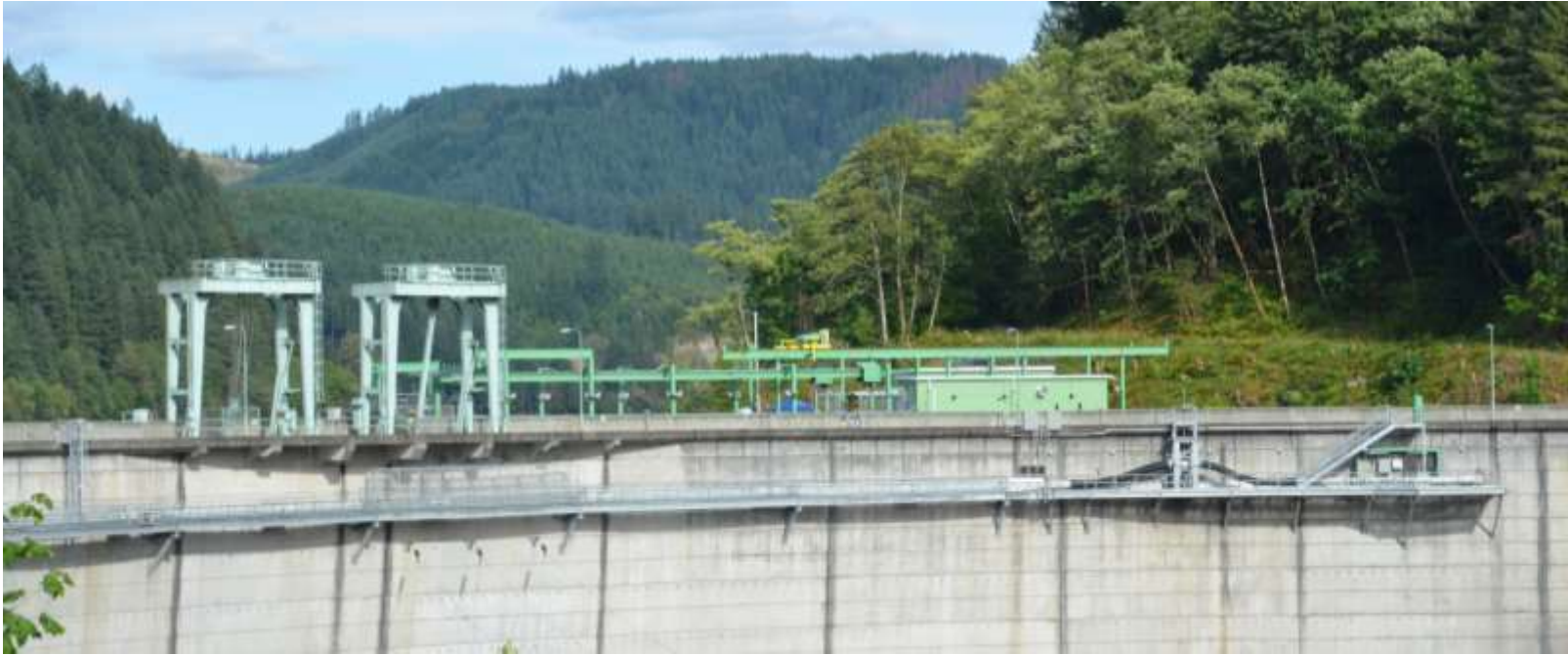
Transport Pipe Along Dam Face
