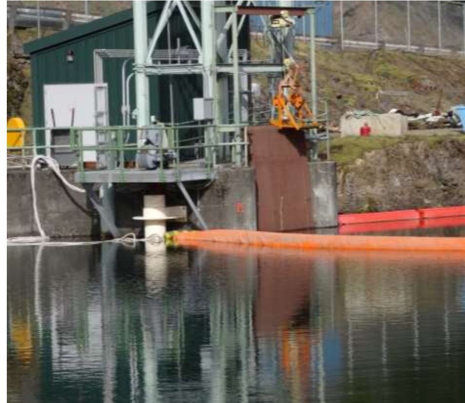
Net Attachment Adjacent to Collector Entrance
