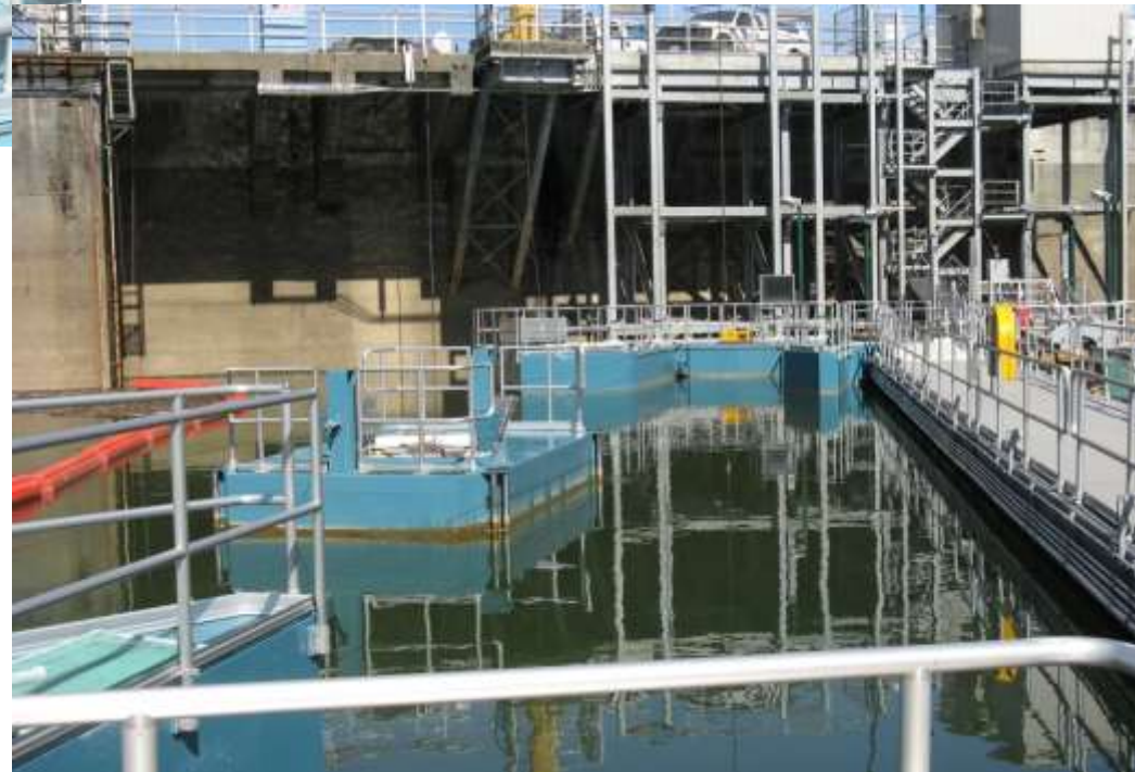
Tanks Barged to Dam for Lifting up to Trucks
