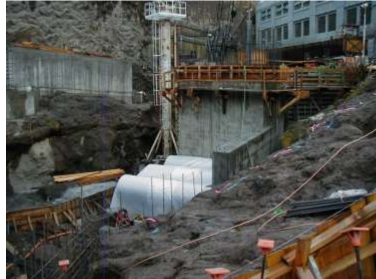
Three T-Screens being Installed
