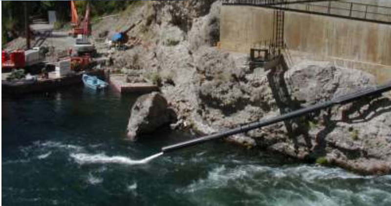
Downstream Bypass Discharge
