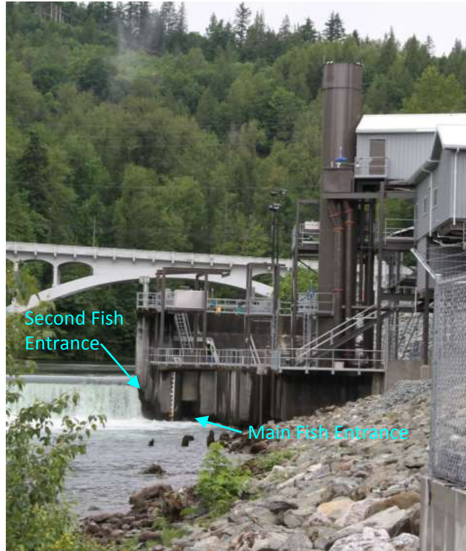
New Fish Lock Facility from Downstream
