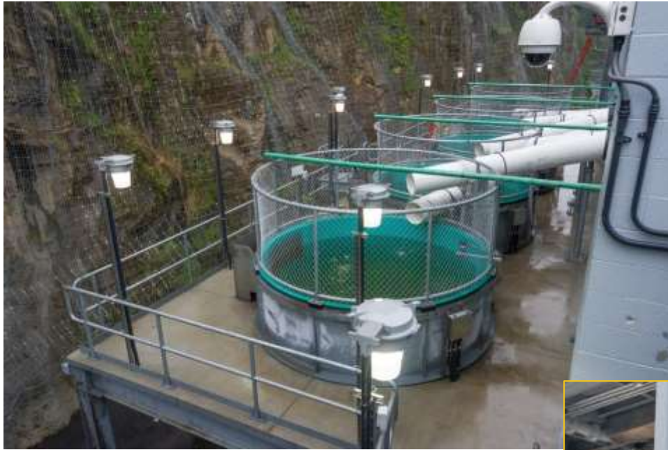
Fish Holding Tanks for Transfer to Transport Trucks
