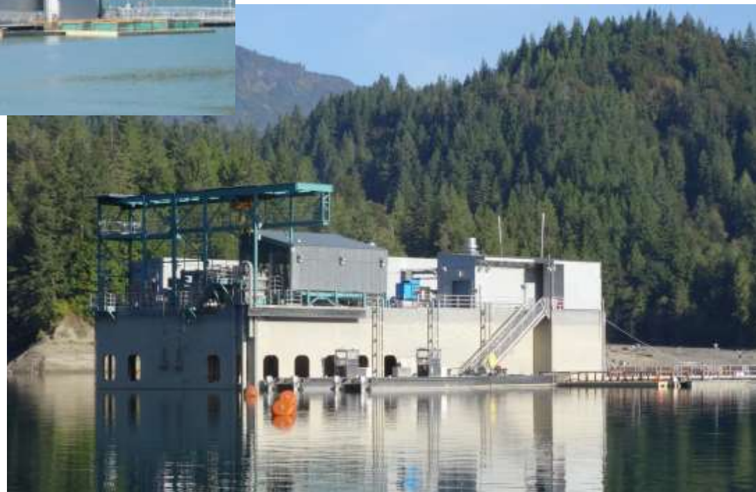
FSC in Un-Ballasted Maintenance Position
