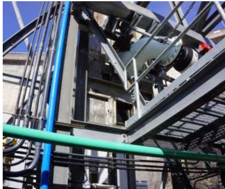
Hopper at Top of Tower Discharging to Conveyance Pipe
